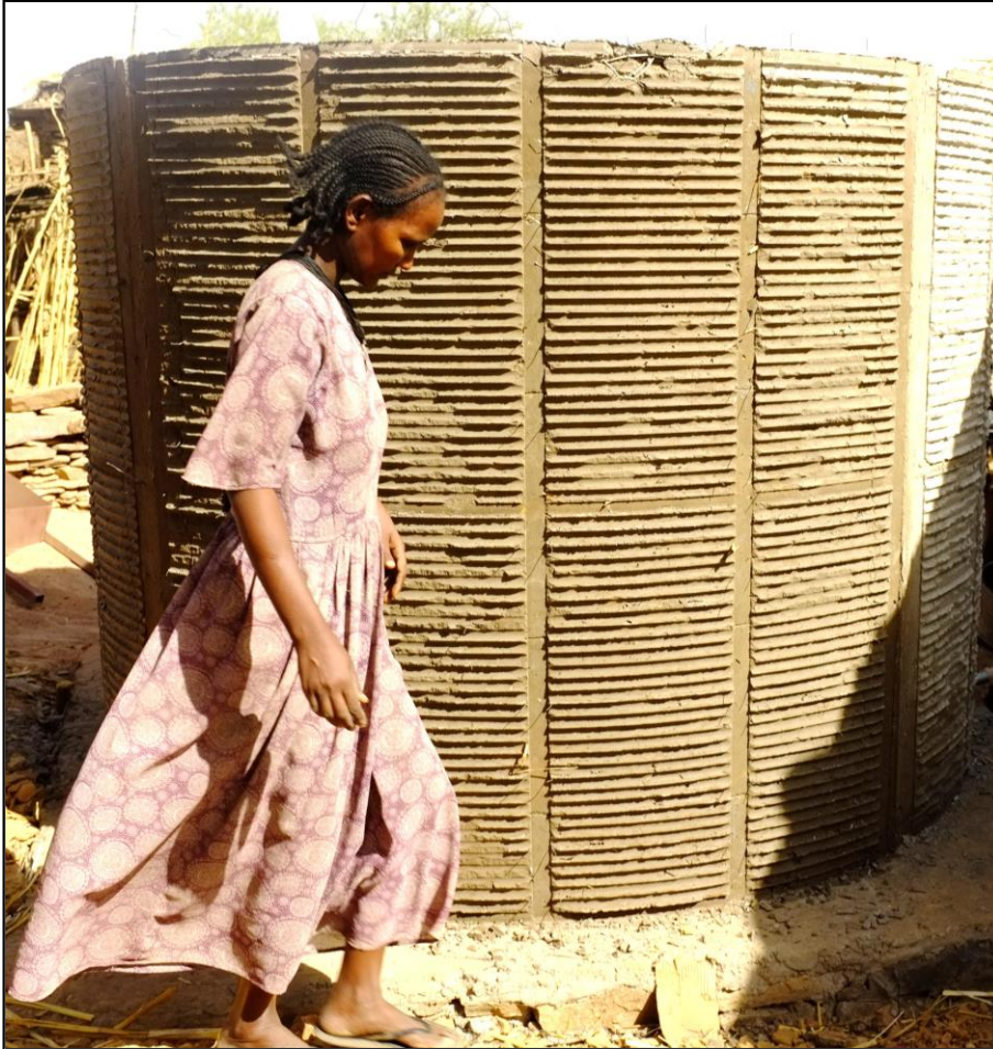
Picture 17: Profile of cistern body after removing the mold
