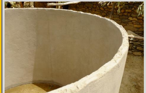
Picture 20: The 7-8 cm thin cistern body after final plastering
