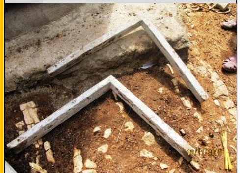
Picture 8: Manhole mold rectangles
