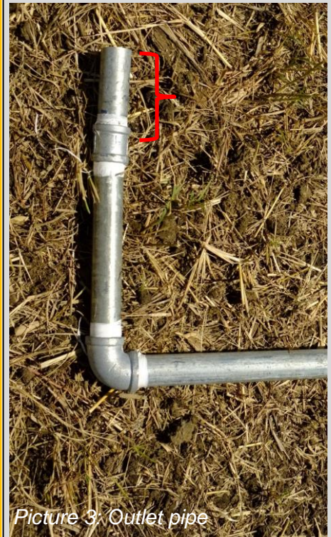
Figure 6: Additional 10 cm concrete floor (marked yellow) will be cast (1) inside the cistern once the cistern body is in place (see Picture 18). A 5 cm section of outlet pipe (marked red) can be detached for flushing out cleaning water.
