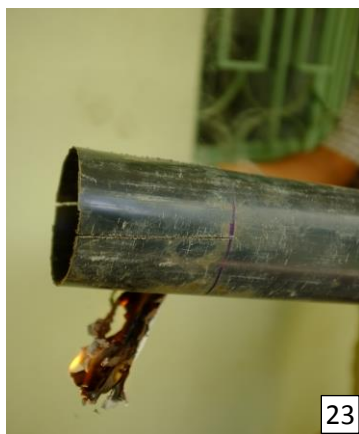
Pictures 21-24: Preparing the cistern cover inlet pipe
