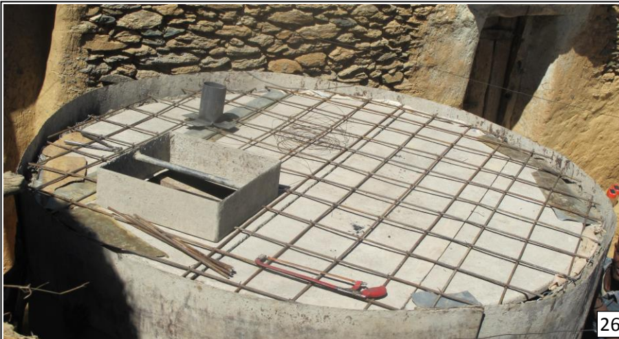
Picture 26: Placing the metal sheet collar and cover mold
