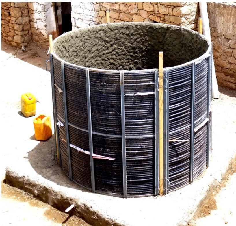
Picture 16: Assembled cistern body mold with one layer cement plastering inside
