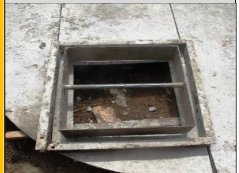
Picture 9: Manhole mold assembled
