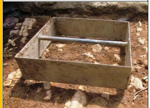
Picture 7: Manhole mold box
