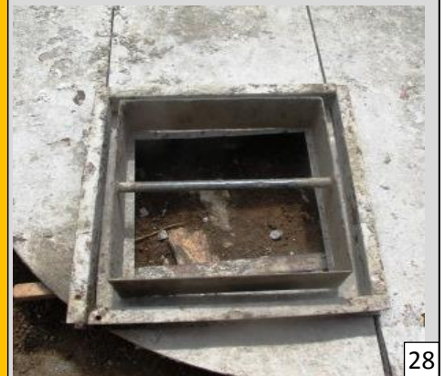
Picture 30: Note: Seal inside manhole lid with a sponge sheet to prevent insects from entering the cistern.
