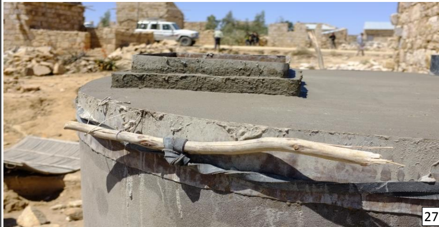
Picture 26: Placing the metal sheet collar and cover mold
