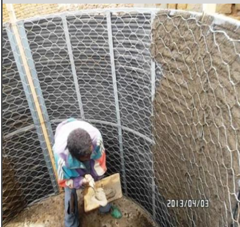
Picture 14: 1 st round cement plastering after lining the wire mesh
