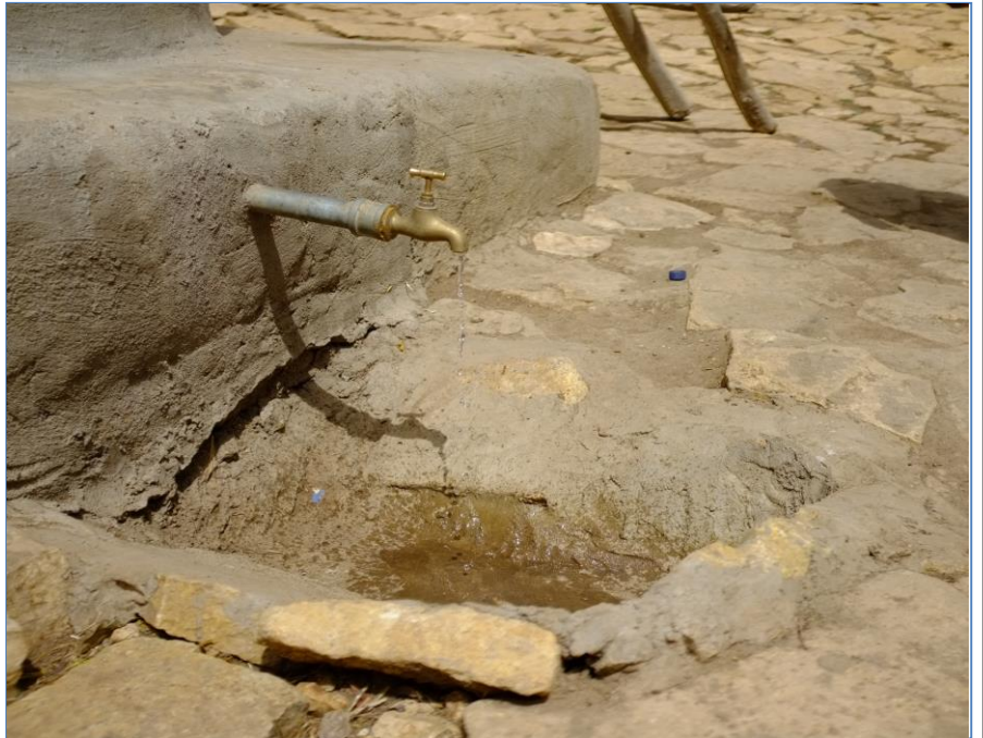
Picture 31: Water outlet pit
