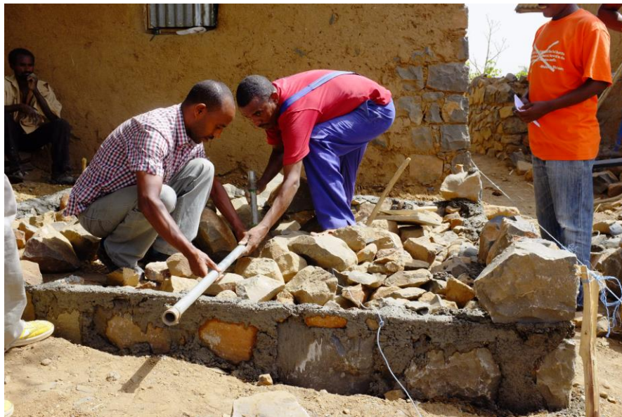
Picture 4: Placing the outlet pipe inside the foundation
