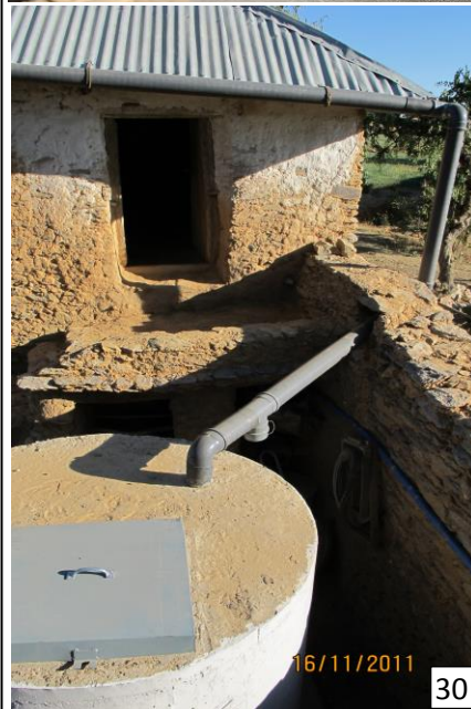
Pictures 27-30: Cistern cover after concrete casting with metal sheet collar mold still in place (27). Placing the manhole molds (28). Manhole after removing molds (29). Manhole covered with lid (30).
