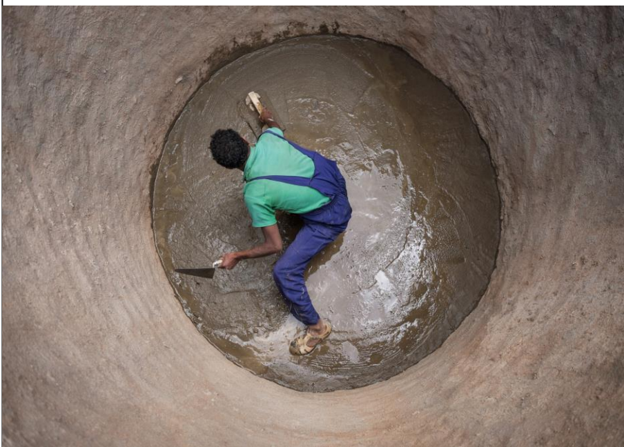
Picture 18: Casting of 10 cm cistern floor after cistern body construction
